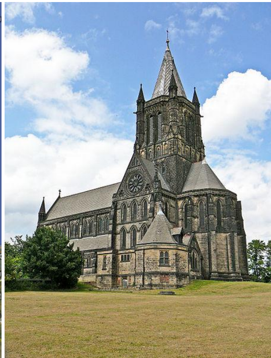
St Bartholomew's Church in Armley
